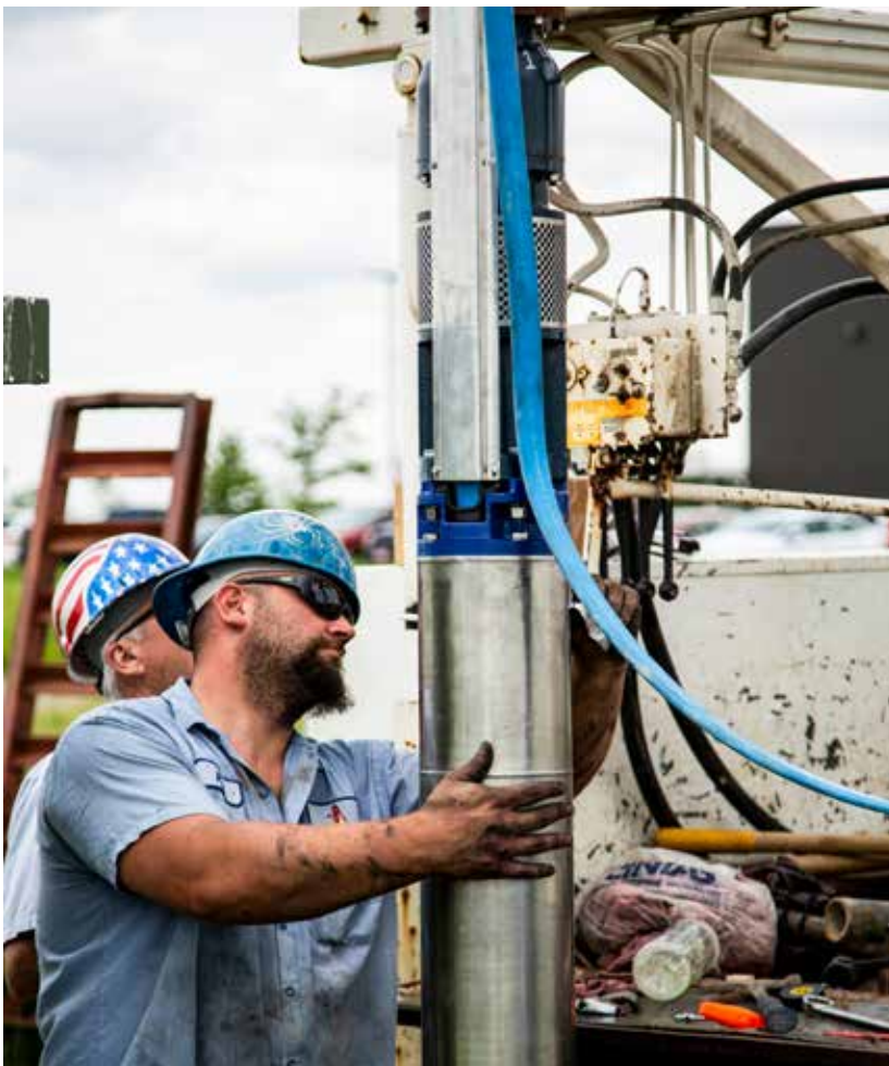
IMAGE 1: Well replacement (Images courtesy of Franklin Electric)
